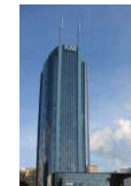
I&M Bank Tower
